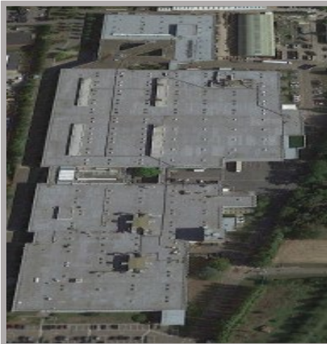
Figuur 1 Commscope Connectivity Kessel-Lo
