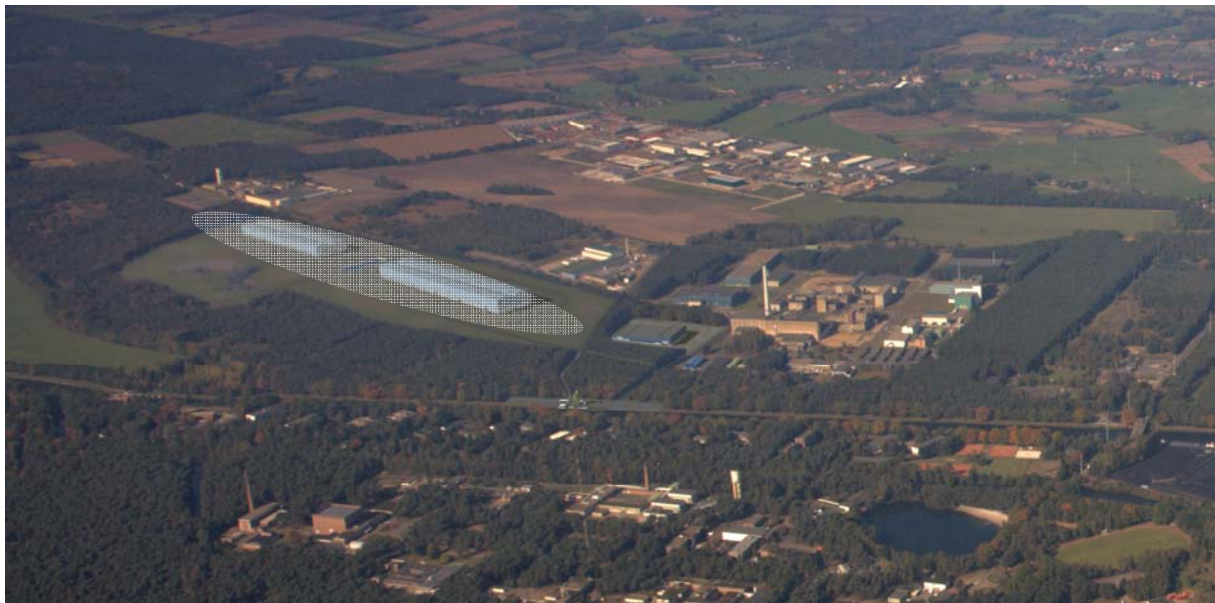
Figure 1: Global view on the future disposal facility (during the operational period) implanted on the Dessel site near to Belgoprocess.
