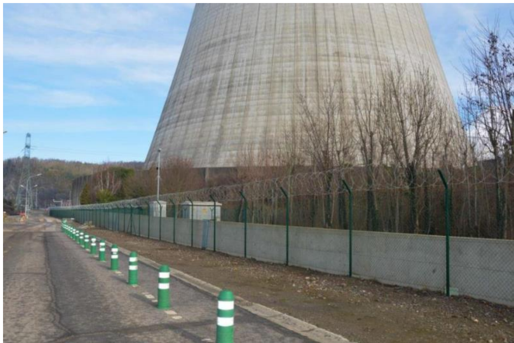
Figure 16 : New peripheral protection of the site of Tihange
