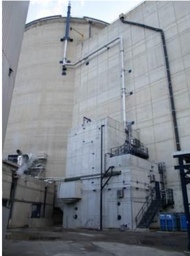
Figure 3: Filtered containment venting system of Tihange 3
